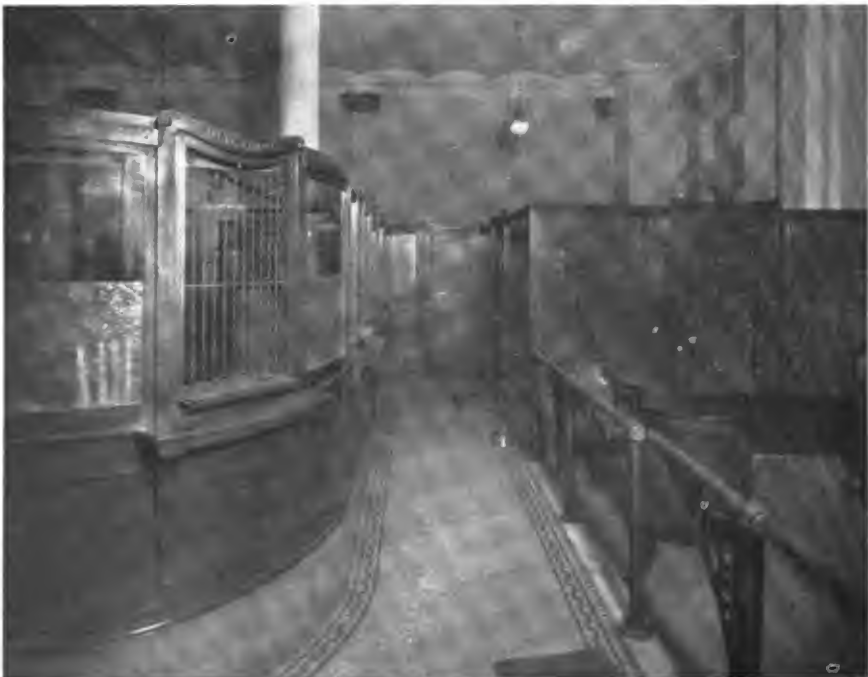
View of Corridor leading to Board Room.
